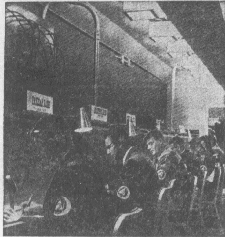
CONTROL CENTER for civil defense in northeastern Illinois near Wheaton, Ill., is an outstanding example of new facilities being constructed to provide city and State governments with headquarters for emergency operations in case of nuclear attack. This underground control center is built to withstand a nuclear blast equivalent to 20 million tons of TNT only three miles away. Heart of the center is the radio communications room, partly shown here. (OCDM Photo)
