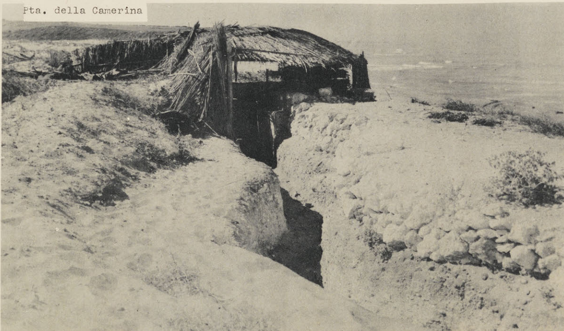
MACHINE GUNS: A camouflaged machine gun position with slit trench. For vertical view see page 14.
