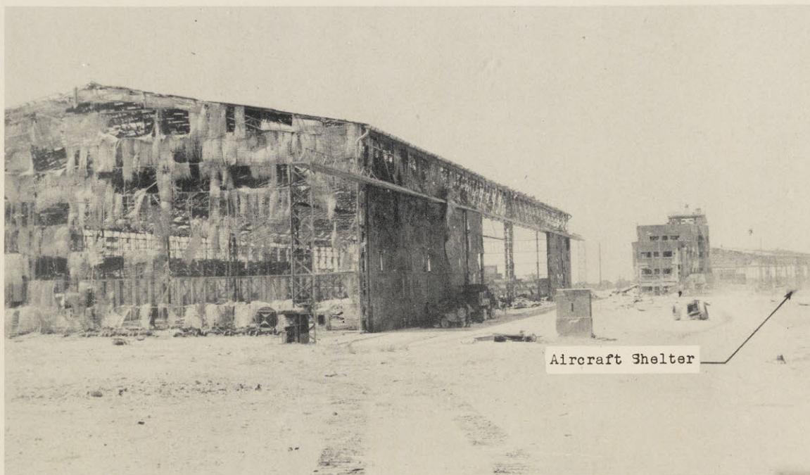
HANGARS : Hangars and control station at the Comiso Airport. For vertical view, see page 31.
