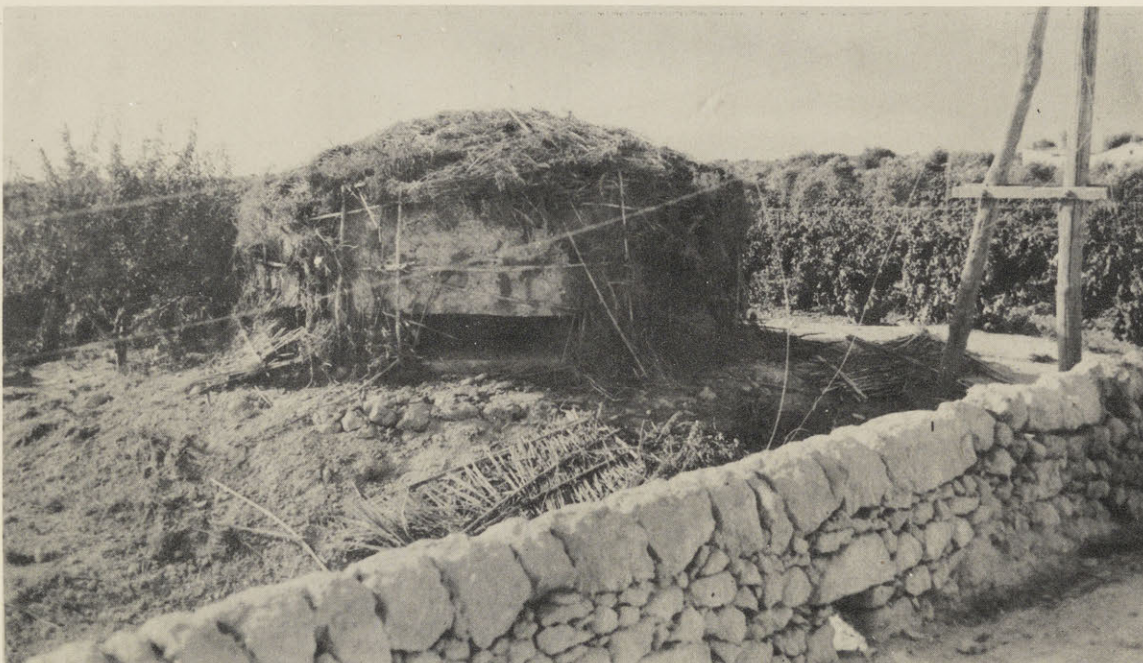
PILL-BOXES : A camouflaged pill-box adjacent to the road blocks within the strong-point on the Scoglitti-Vittoria highway. For vertical view see page 24, and for diagrams, see page 28.
