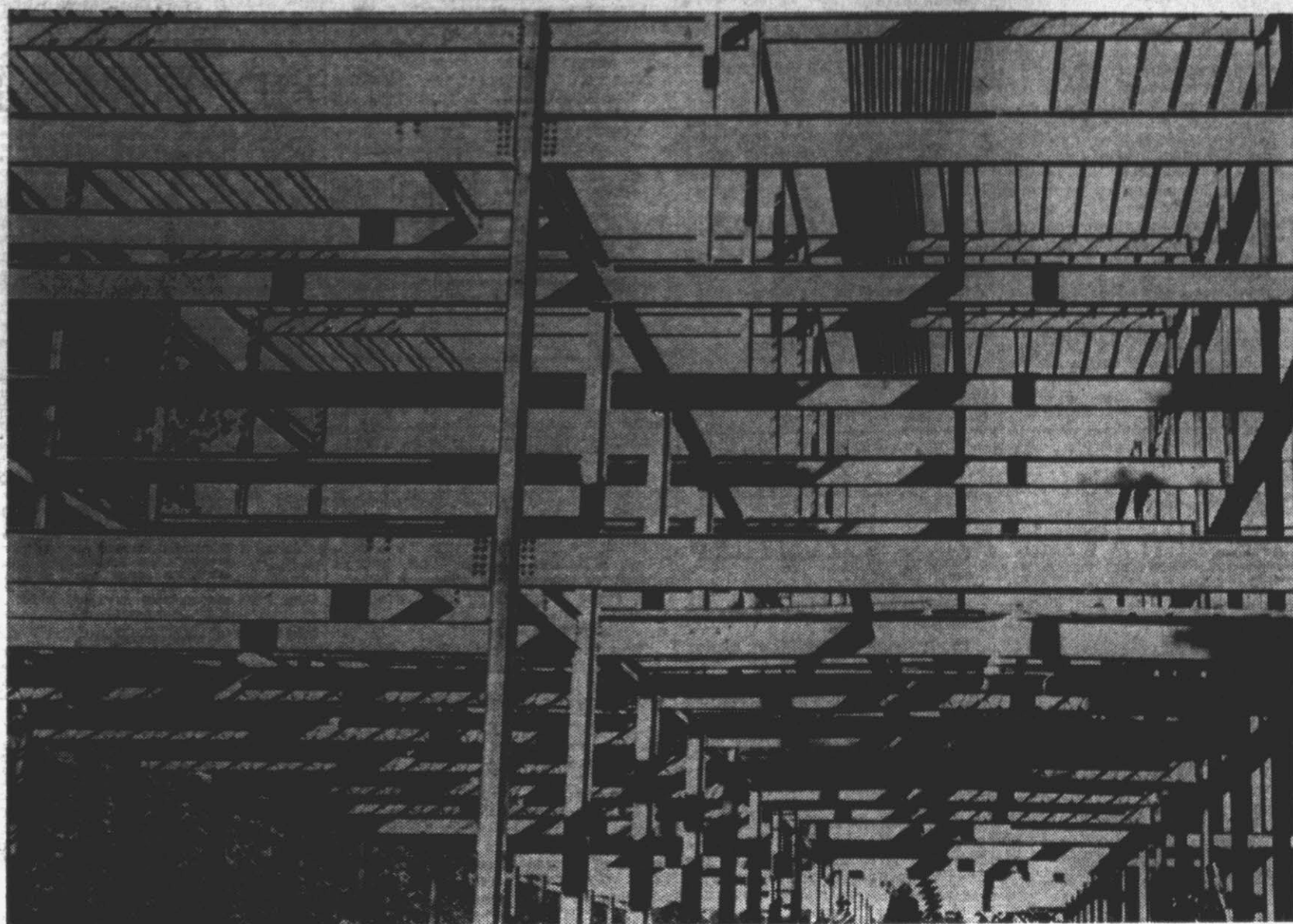
STEEL RISES FOR ECC'S NEW CLASSROOM BUILDING... part of nearly $3½ million in new construction for city this year.
