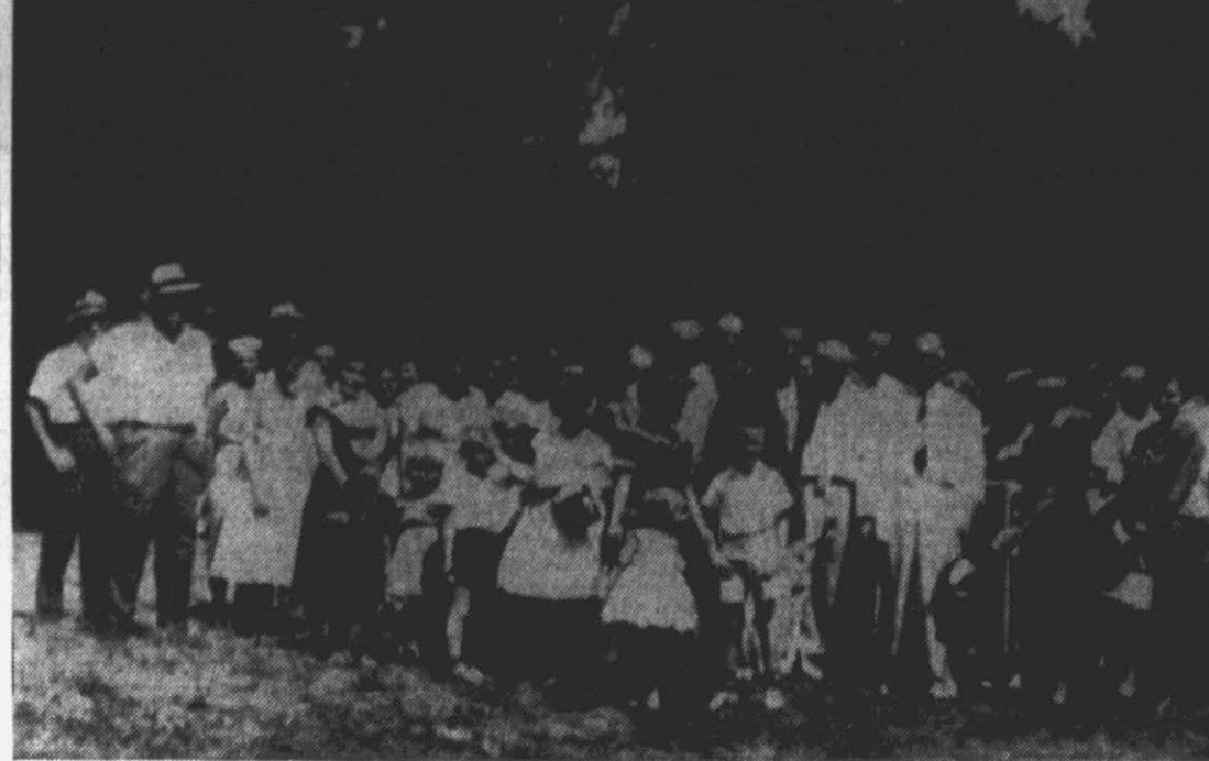
BUILDING A PARSONAGE.—Ground was broken last Sunday for a new parsonage at the Mount Pleasant Christian Church. A large number of the congregation was in attendance for the ceremony. The first shovelful of earth was turned by Mrs. Rosa Briley.
