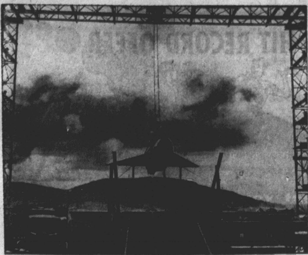
STEP BY STEP TESTING —The Short SC1 vertical takeoff and landing research aircraft rises in its test gantry during hovering tests at Belfast, Ireland. Gantry tests will continue before craft makes a free vertical takeoff followed by forward flight.
