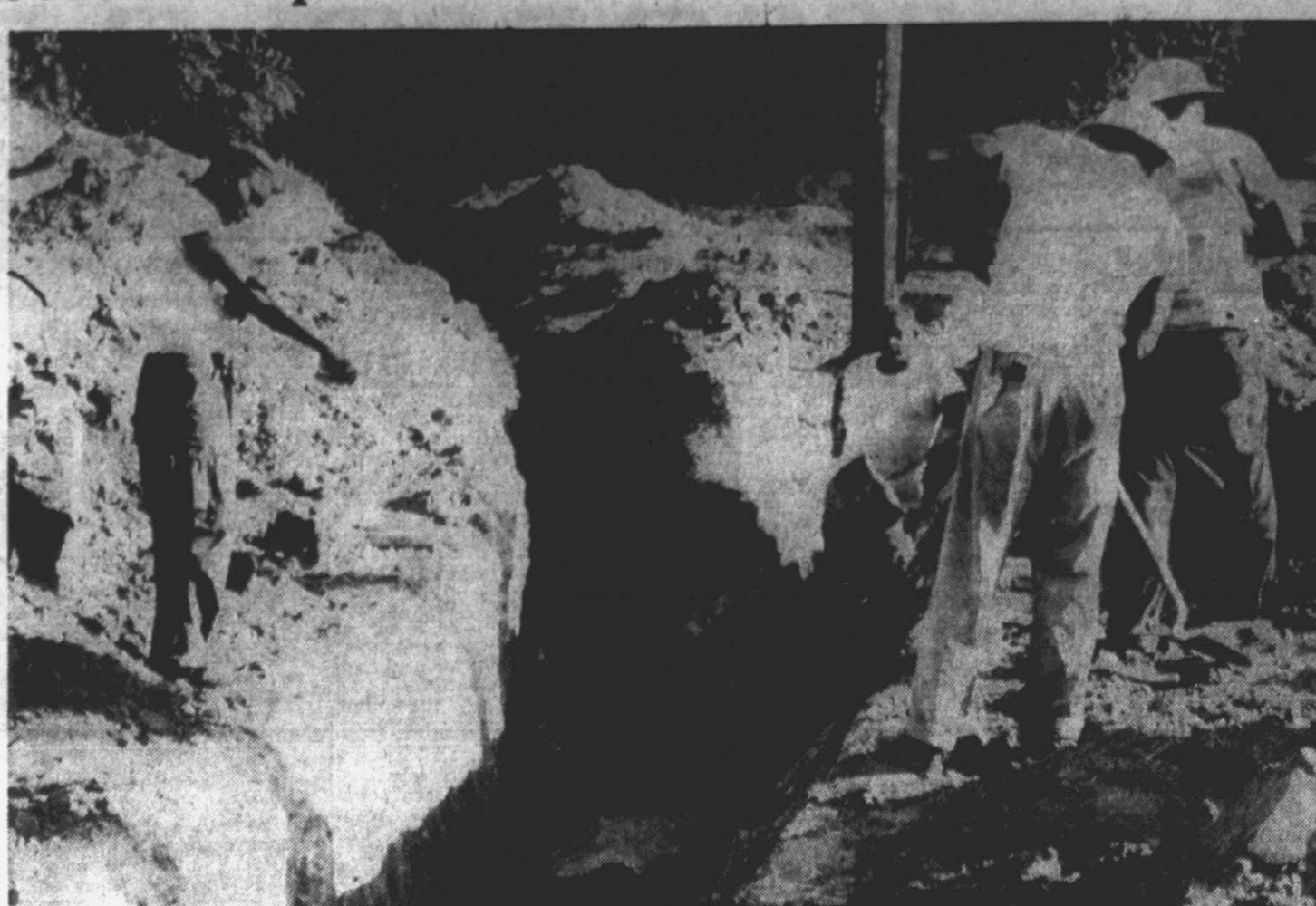
WORK NEARING COMPLETION ON NEW STEAM LINES . . . For East Carolina College's New Dormitory South Of Tenth Street
