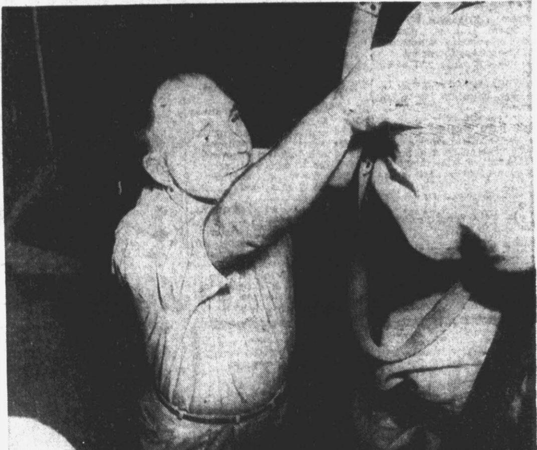
ROSE HIGH DRILLS . . . Light equipment first
