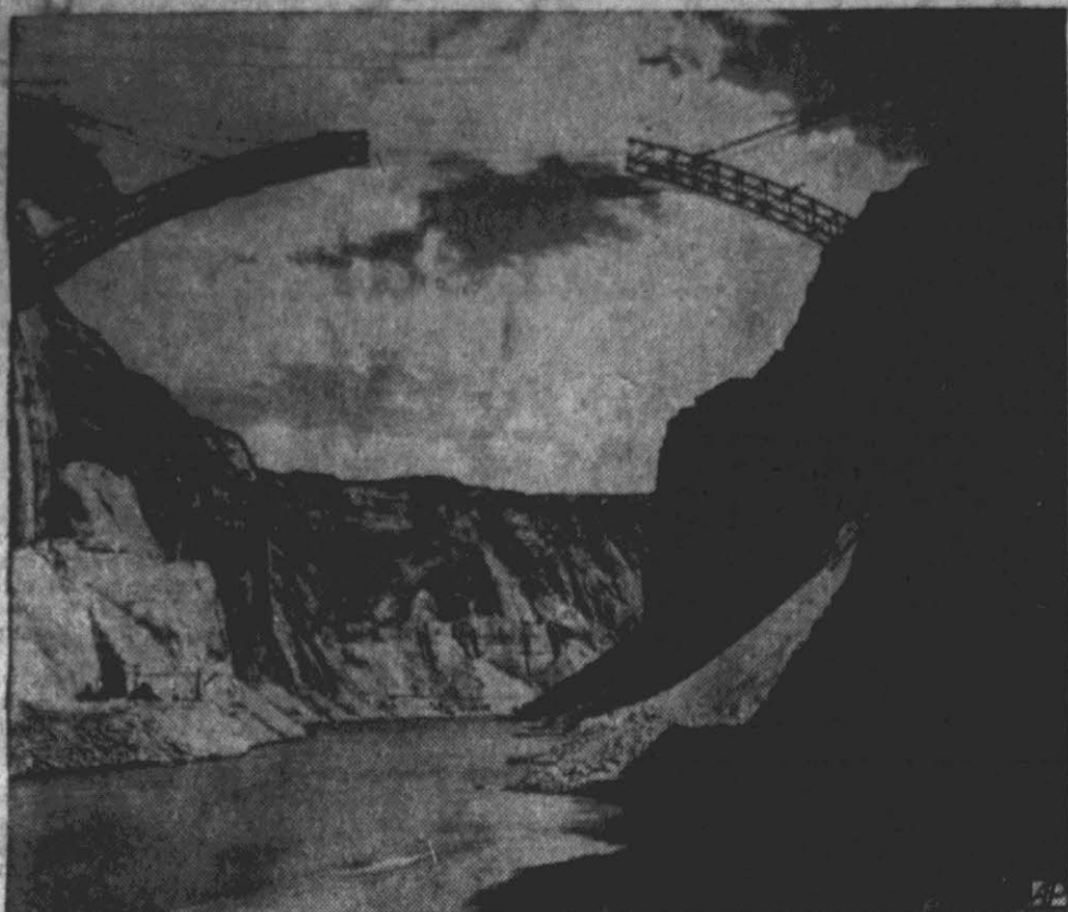
SPANNING THE COLORADO — Work on a steel arch bridge near completion 700 feet above the Colorado river near Glen Canyon Dam in northern Arizona. The 1,928-foot long bridge, to carry auto traffic, will be only one along 300-mile stretch.
