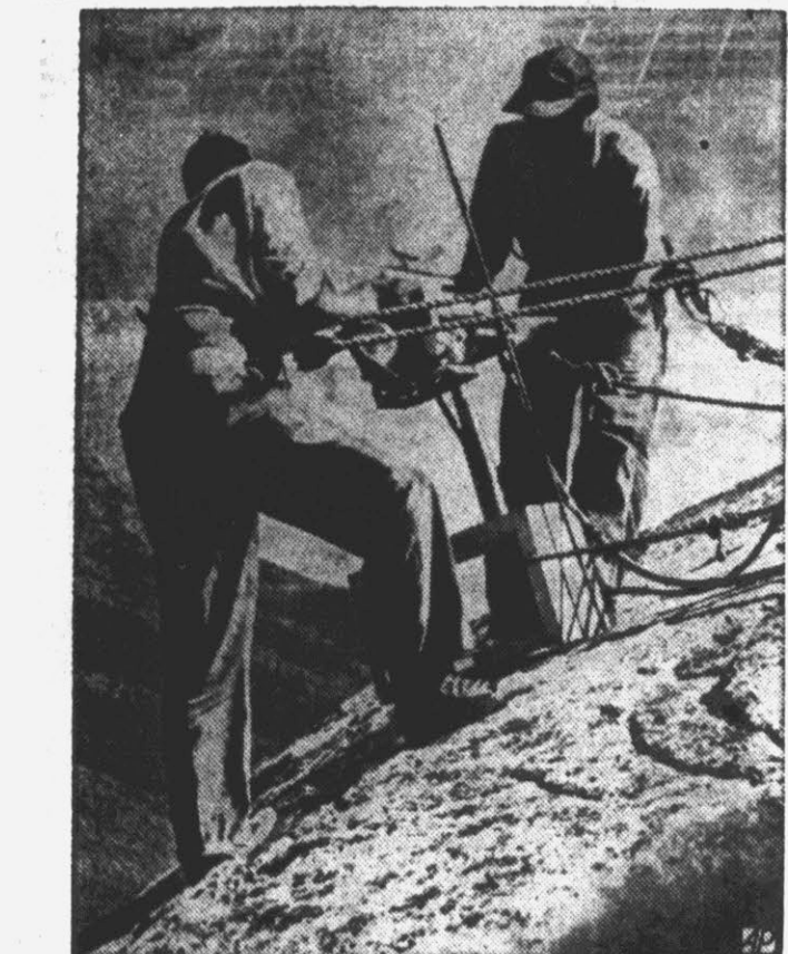
'FACE' SAVING — Workers drill holes for U-belts and turnbuckles to hold stones that form historic profile of "Old Man of the Mountain" at Franconia, N. H. Nature weakened the "face" and man is trying to save it.
