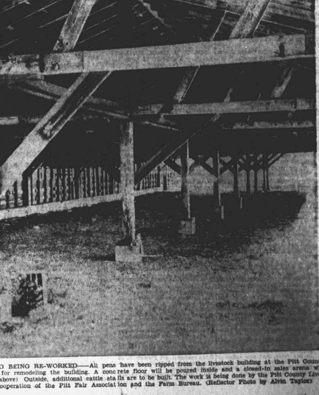
LIVESTOCK BUILDING BEING RE-WORKED—All pens have been ripped from the livestock building at the Pitt County Fair grounds in preparation for remodeling the building.
