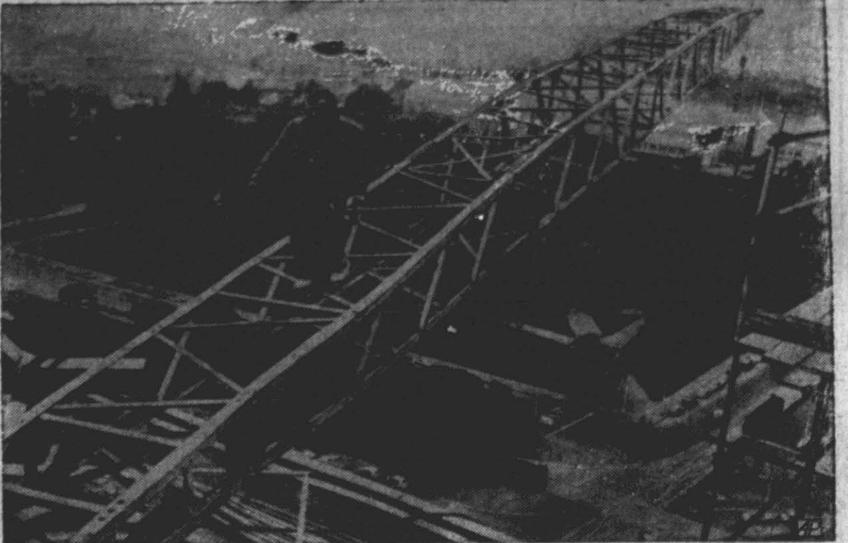
STEP BY NERVY STEP — Gerrit Mulder moves carefully on his job as oiler on crane 250 feet in air during the construction of a 19-story building in Melbourne, Australia.
