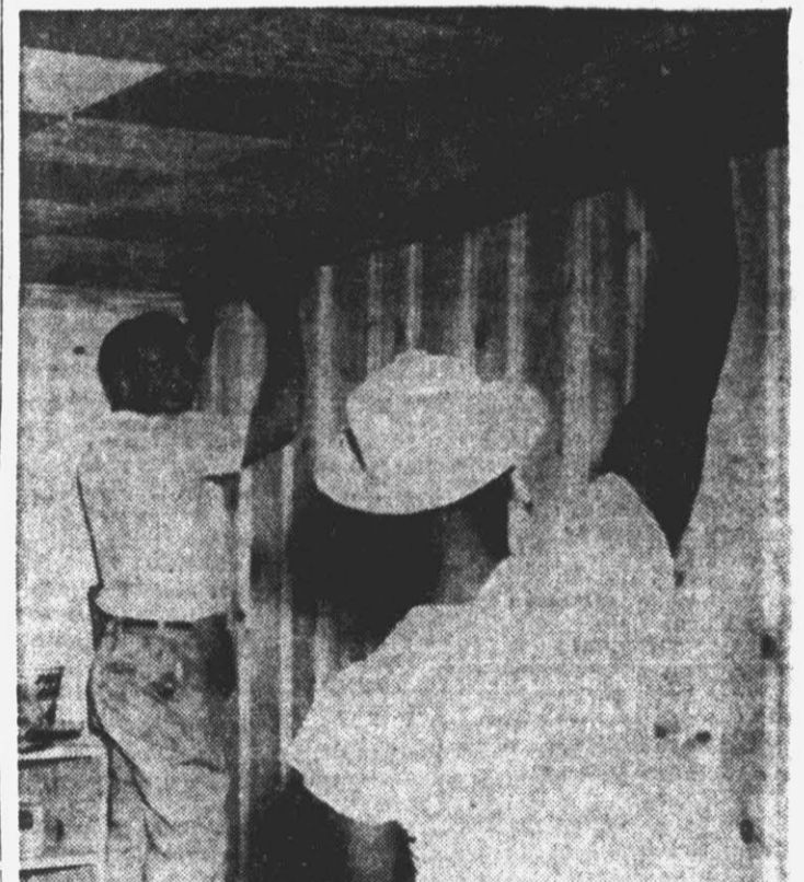
WORKERS IN PRO SHOP... renovation to be completed around September 1.
