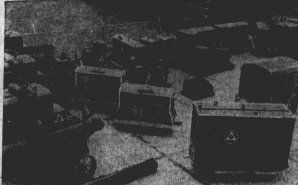
TYPICAL UNIT of civil defense stockpiled engineering equipment showing the pumps, generators, water purifiers, and some of the miles of flexible-coupled pipe which could be used after an attack to provide a stricken community with pure water. Some of this "hardware," grouped in "Ten-Mile Units" to service ten miles of pipe each, already has been used in natural disasters to pump out flooded areas, and to bring in and purify water for towns with dry reservoirs. (ODCM Photo)
