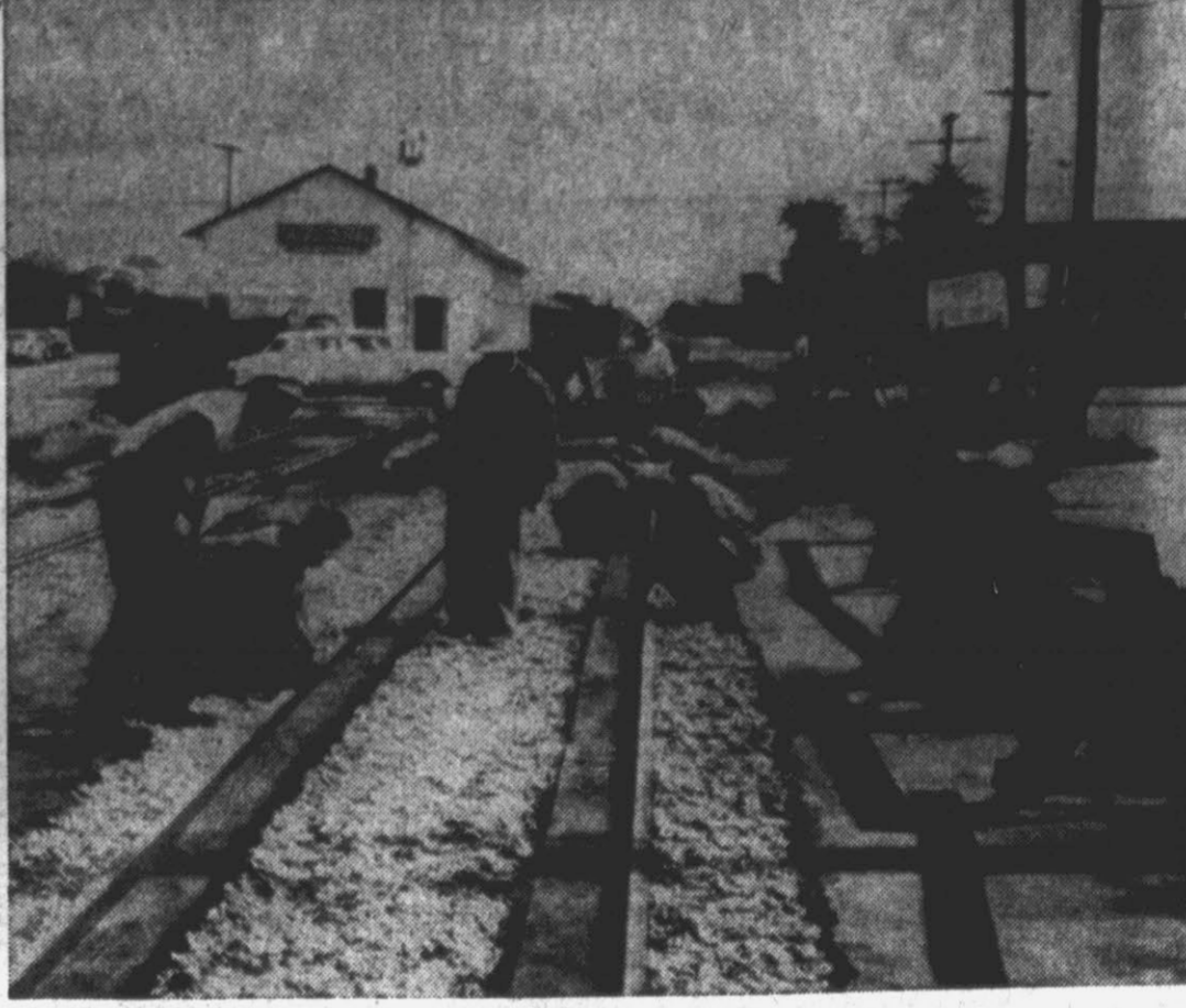
ATLANTIC COAST LINE REPAIRS CROSSING . . . Dickinson Ave. crossing is re-worked.
