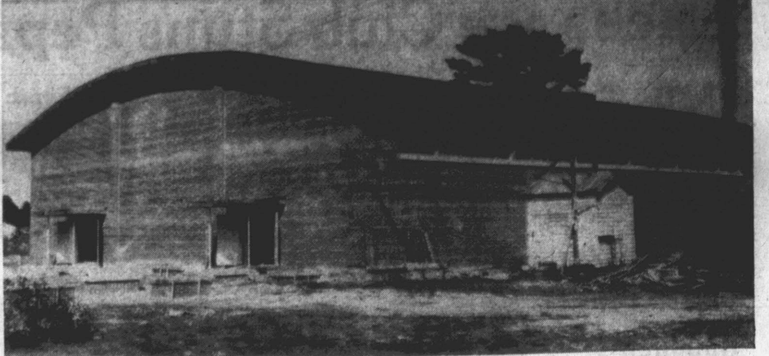
UNDER CONSTRUCTION—Grifton High School's new gymnasium is currently under construction and should be ready for use before the beginning of the 1958-59 term. Actual construction began in January but inclement weather hindered workers. The gym, with a seating capacity of approximately 1,000 people, measures 80 feet by 100 feet. In addition to the basketball courts, there are two dressing rooms for each of the boys and girls, storage rooms, a lobby and bathroom facilities for both men and women. (Reflector Photo)
