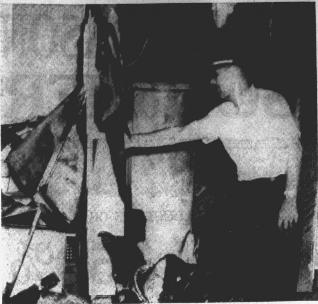
ASSISTANT FIRE CHIEF JASPER JONES... looks over damaged dwelling.
