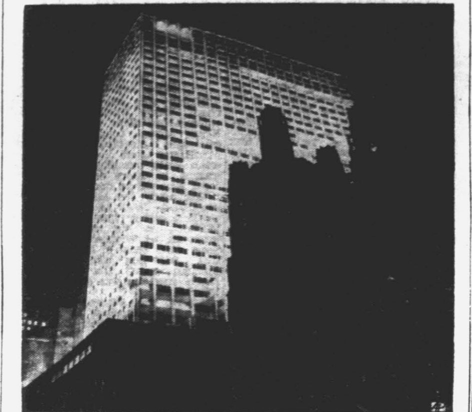
SKY LIGHTER — Beams from reflector lamps brighten the aluminum facade of the new 39-story Tishman building on Manhattan's Fifth Avenue. At lower right is St. Thomas Church.
