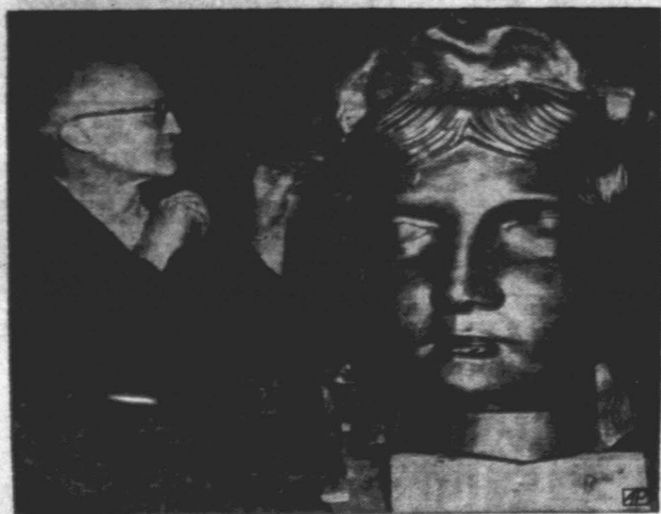
HEADING EAST — Workman completes head of Victory goddess, part of West Berlin's contribution to war-damaged Brandenburg Gate being restored in East Berlin section of city.
