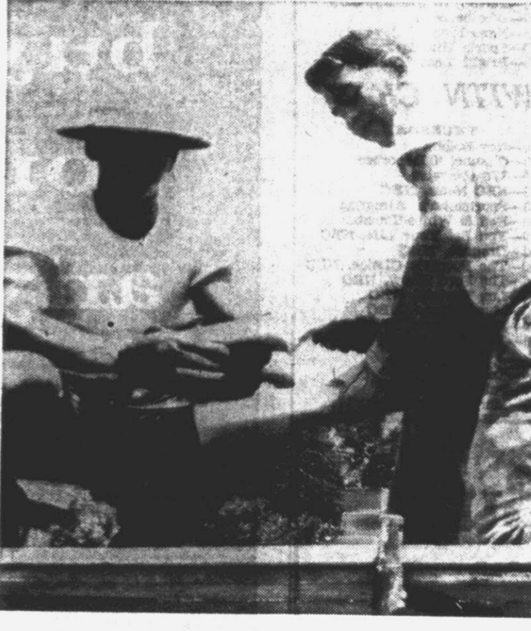
CONSTRUCTION WORK ... Bill Clapp and Nat Van Nortwick are employed by the North State Construction Company. They are helping construct buildings at ECC.
