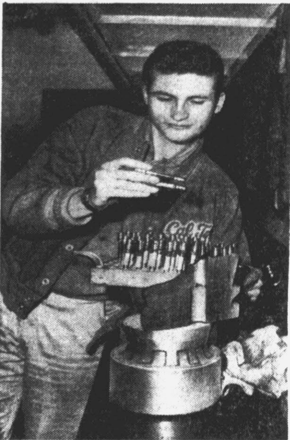
Student Jerry Peck tests metals for metal fatigue. Samples were cut from wind-tunnel propeller hubs.
