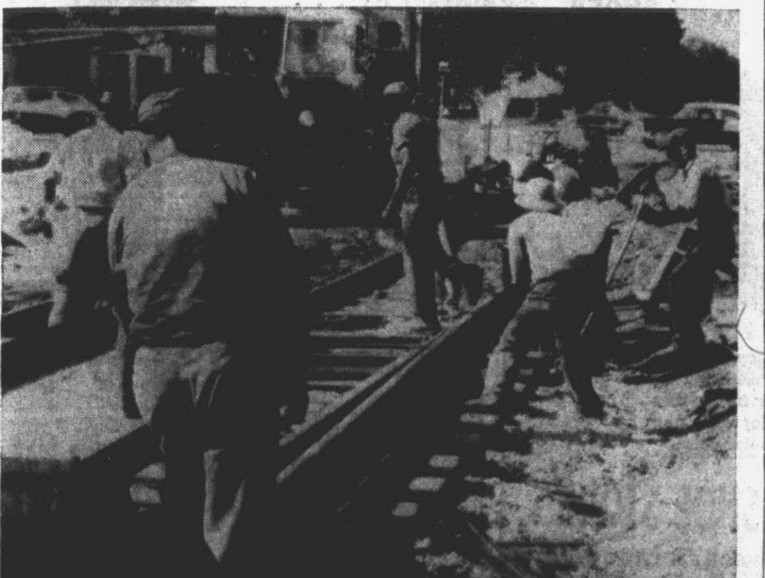
CROSSINGS REPAIRED . . . ACL rehabilitates lines through Greenville.
