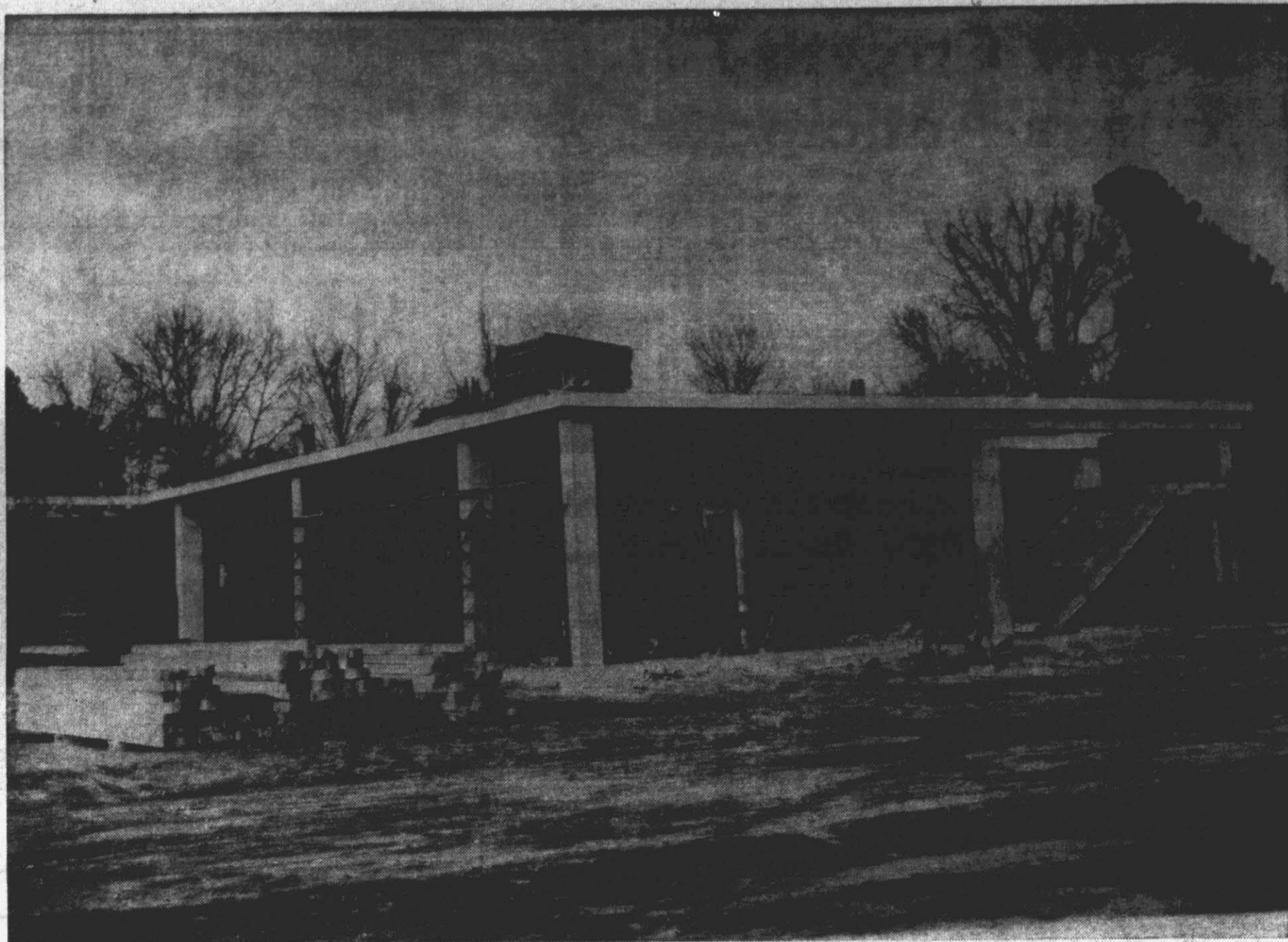
New Men's Dormitory Under Construction
