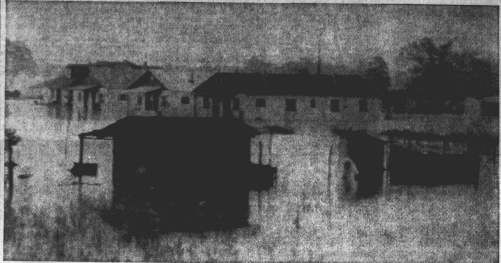
TAR ENGULFS HOUSE ON NORTH SIDE . . . 30 dwellings affected by flood
