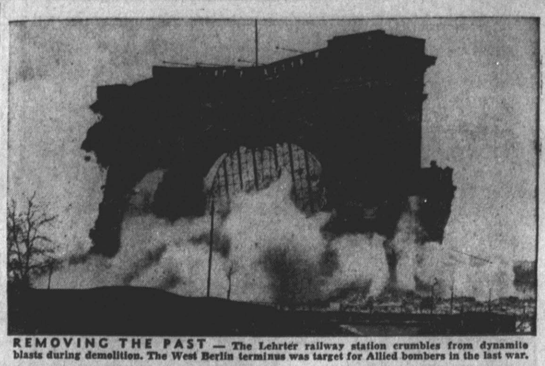
REMOVING THE PAST — The Lehrter railway station crumbles from dynamite blasts during demolition. The West Berlin terminus was target for Allied bombers in the last war.
