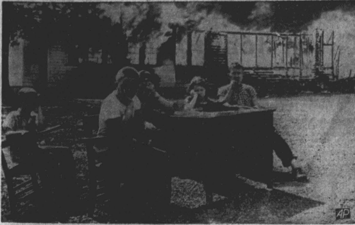
SCHOOL BURNS—Fire destroying the public school in the Adamsburg community near Fort Payne, Ala., attracted these youngsters to the grounds to watch but they ended up sitting in the only furniture saved from the ill-fated building. There'll be no more school in this building, and all but the little fellow at left seem sad. (AP Wirephoto)
