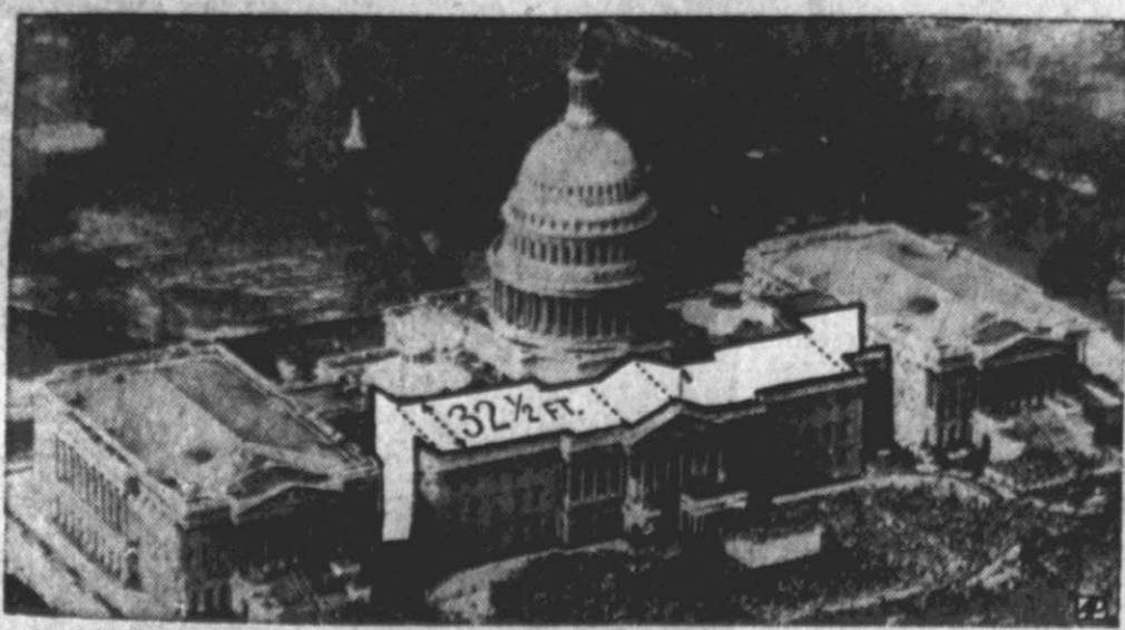
WHAT'S PROPOSED—Altered photograph shows major part of proposed Capitol alteration, which would move present east wall forward 32 1/2 feet. Proponents say it would improve the building's lines and make room for needed additional office space and dining facilities.
