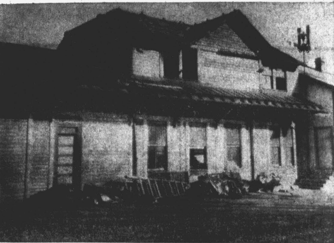
OLD ACL PASSENGER STATION TICKET OFFICE . . . building is being torn down. (Reflector Photo).
