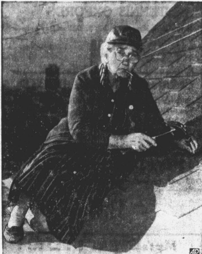
NEVER TOO OLD—Roofing is all in the day's work for Mrs. Verdie Scott of Midland, Tex. The 75-year-old widow does roof repairs, electrical work and is a licensed plumber.
