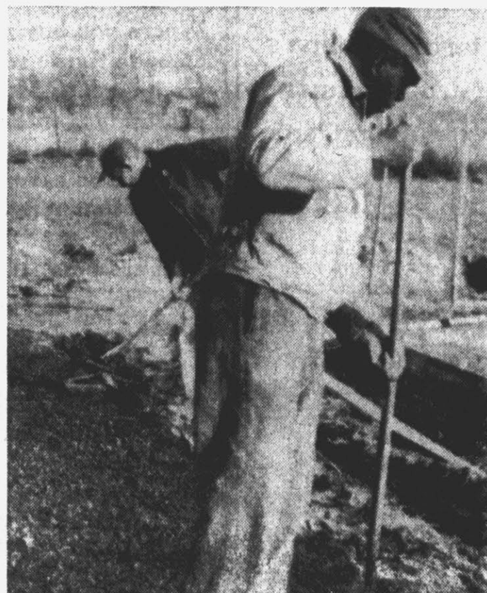
WORKER LEVELS OFF THE SOIL . . . bed should be level for drainage.
