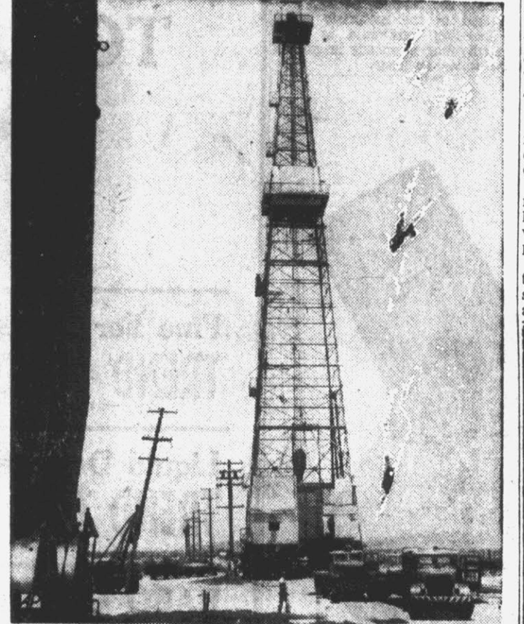
THE BIG TRANSFER — A sight not seen by many is a giant oil derrick on the move. Here's one being hauled by structural movers to new location at Huntington Beach, Calif.
