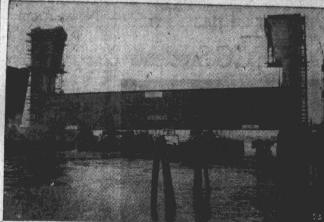
FLOOD WATER CONTROL — Giant steel door is positioned between towers on the Hollandse Yssel river near Rotterdam. Door will be lowered when high tides threaten the area.
