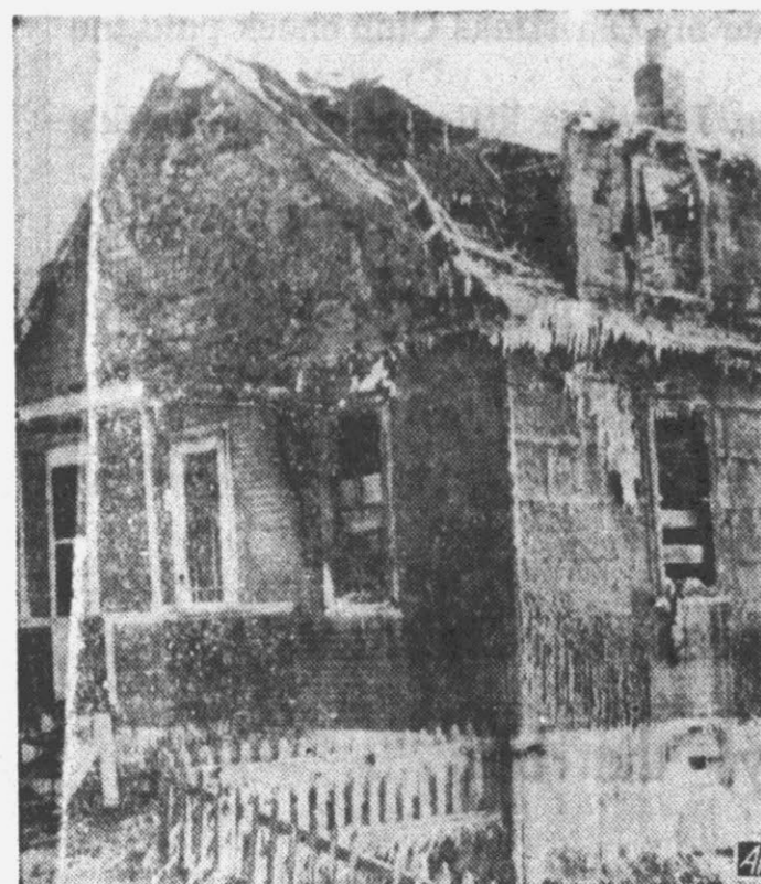
WHERE 8 CHILDREN DIED:—This is the fire-gutted, ice-covered home of Liorel Denault on the outskirts of Sherbrooke, Quebec, in which 8 children were trapped by fire and perished.
