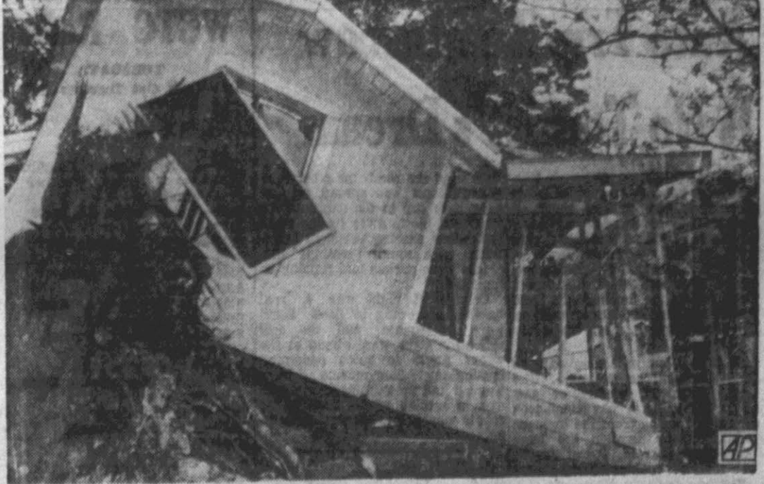
STORM STRIKES SOUTHERN CALIFORNIA:—Winds of hurricane force roared out of southern California canyons and left a trail of wreckage in their wake. This house in Tujunga, a Los Angeles suburb, was one of the structures damaged. Part of the building was knocked from its foundation and a corner was lifted five feet high. A large tree at left was uprooted. (AP wirephoto).
