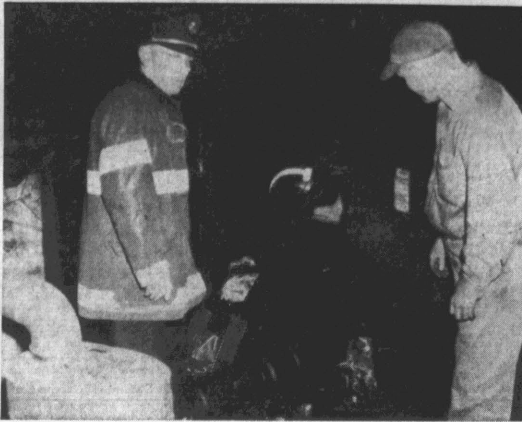
Firemen look over damage which was caused when fire broke out in a dwelling at 713 Fleming St. around 12:30 p.m. yesterday. The house was heavily damaged by the flames. (Reflector Staff Photo.)
