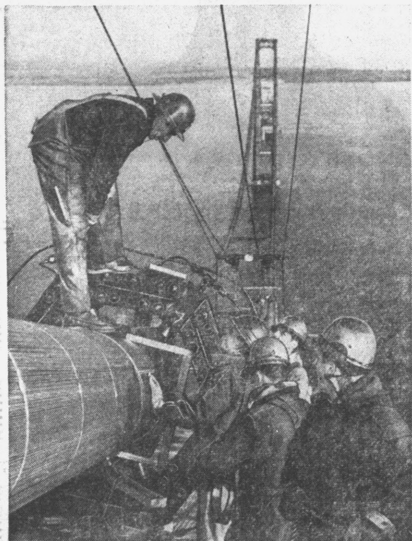
Bridgemen, working high above the Straits, "squeeze" the 12,580 wires of each cable into compact cylindrical mass.
