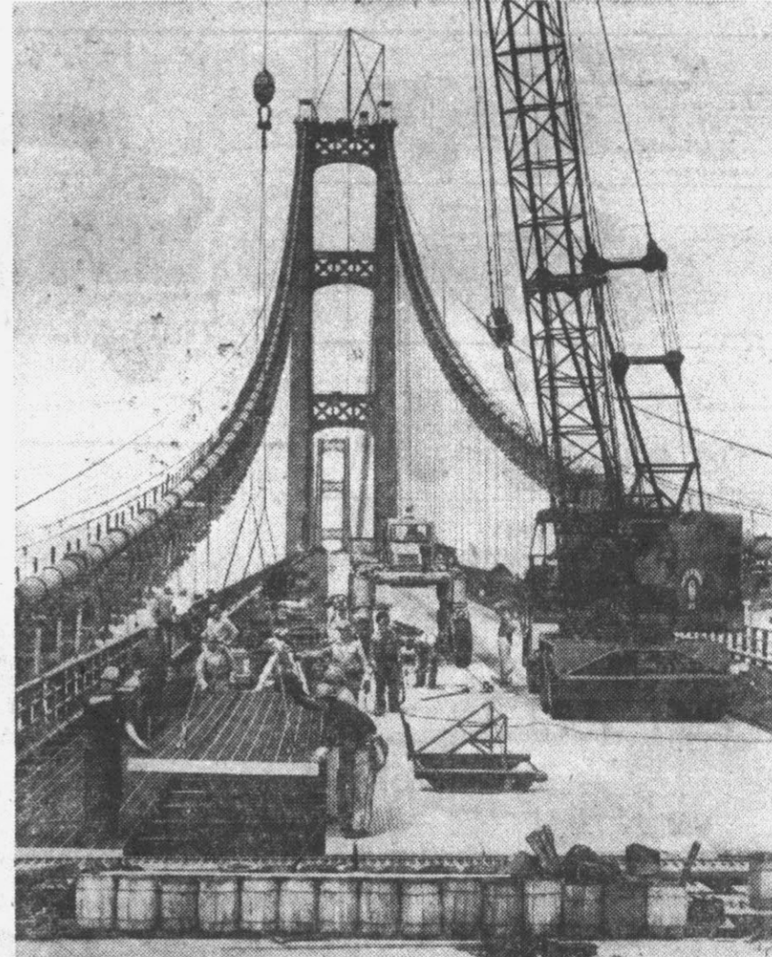
Last steel deck surface section is laid into place.
