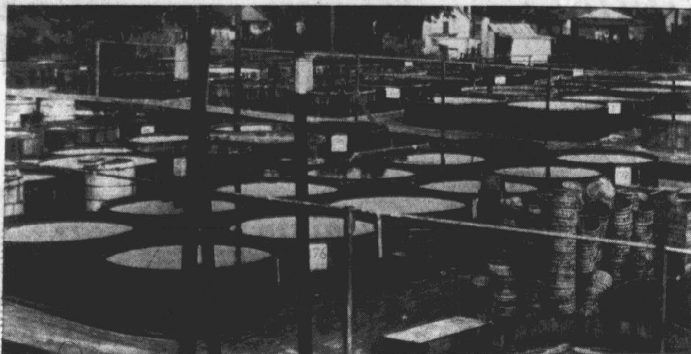
AYDEN PICKLE PLANT'S VAST OUTDOOR CUCUMBER STORAGE FARM ... facilities to store 250,000 bushels of cucumbers in over 1,000,000 gallons of salt brine.
