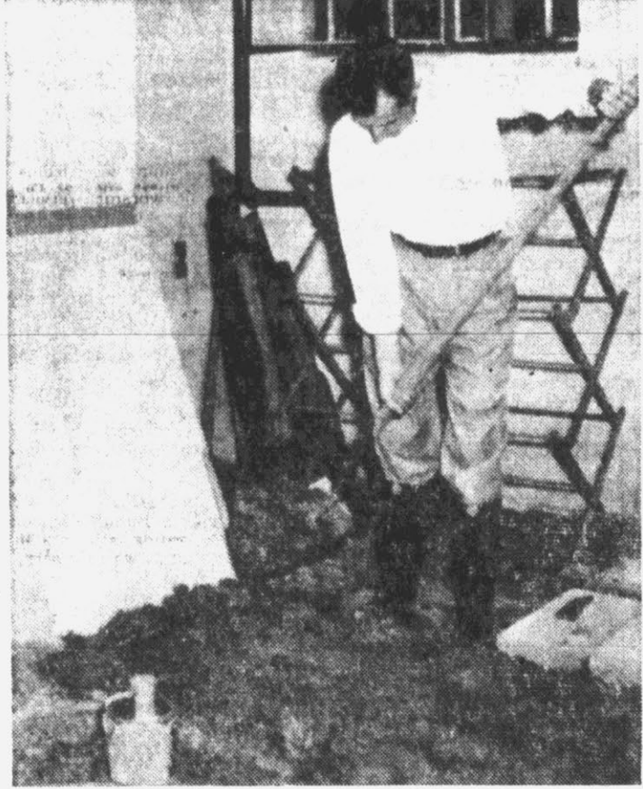
After completing major improvements both in and around his home, he is now busy covering the duct which carries the cool air from an artesian well into his home. The device, which he made himself, completely cools his home.
