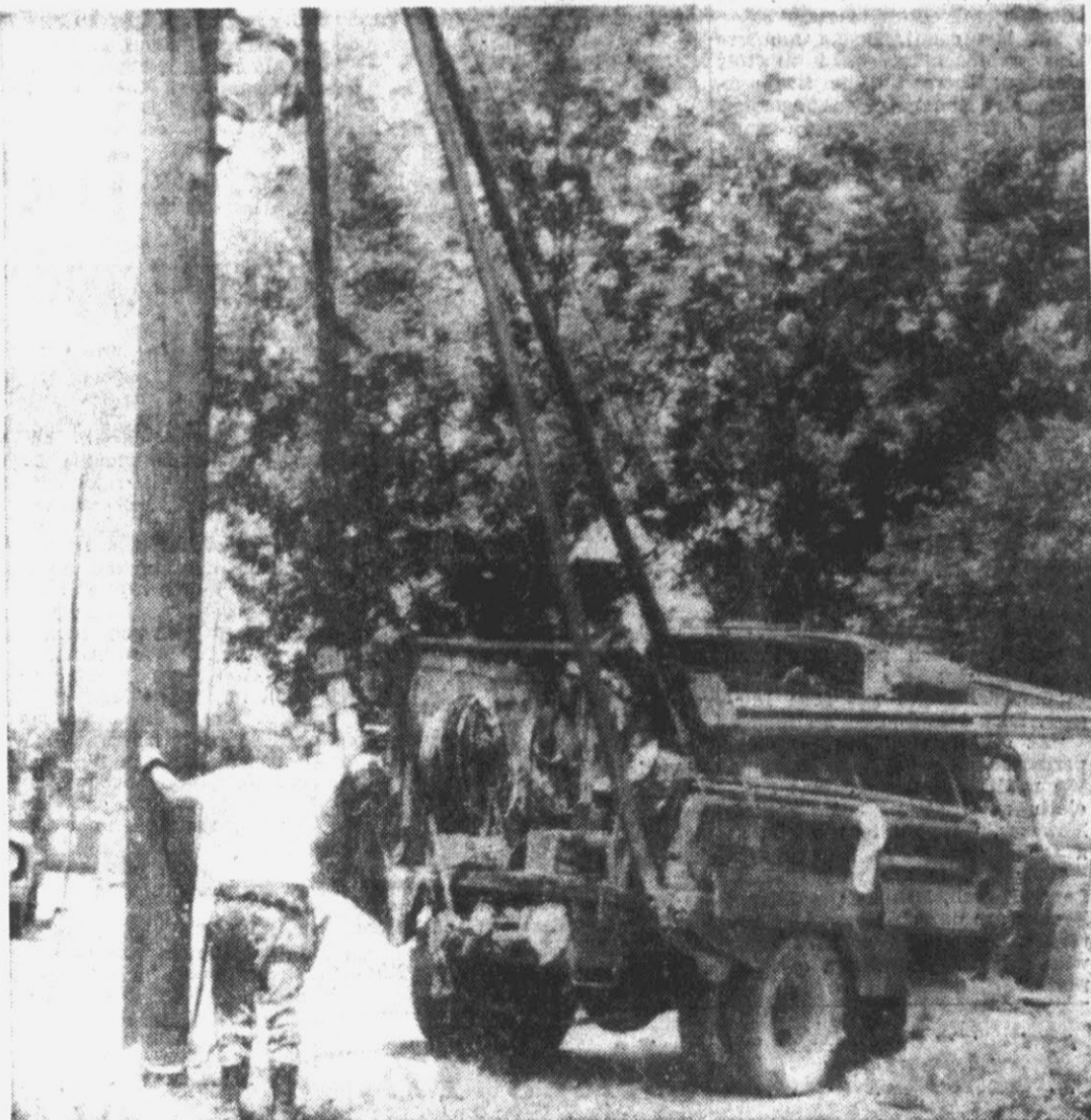
LINING UP . . . the heavy crane is attached to old pole.
