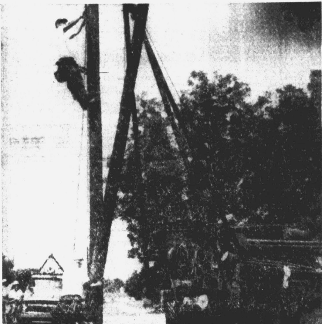
MOVING . . . the pole begins to give.
