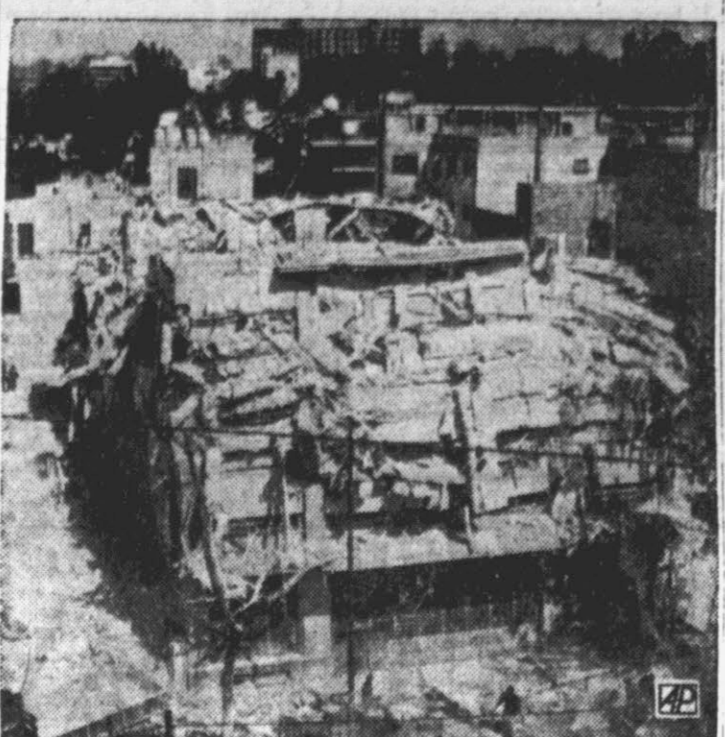
This four-story apartment building collapse in Mexico City in the worst earthquake ever to hit the city. Five persons were believed trapped in the ruins of this building. Over 500 persons have been injured and 52 known dead in 50 toppled buildings in Mexico City alone. The rubble at left covers a dozen cars in parking lot. (AP Wirephoto).
