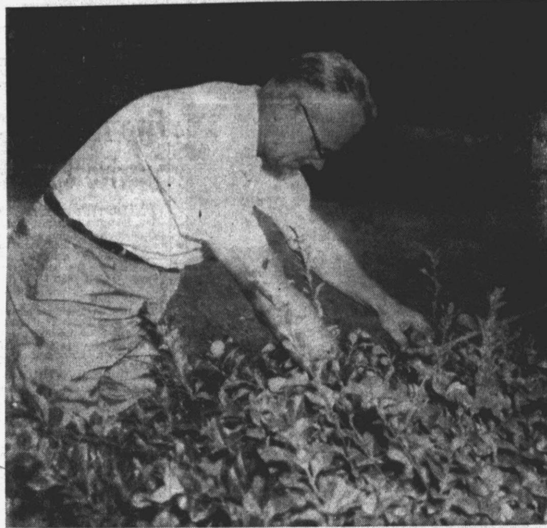
IRRIGATION SYSTEM . . . Hendrix turns on sprinkler head concealed in shrubbery.
