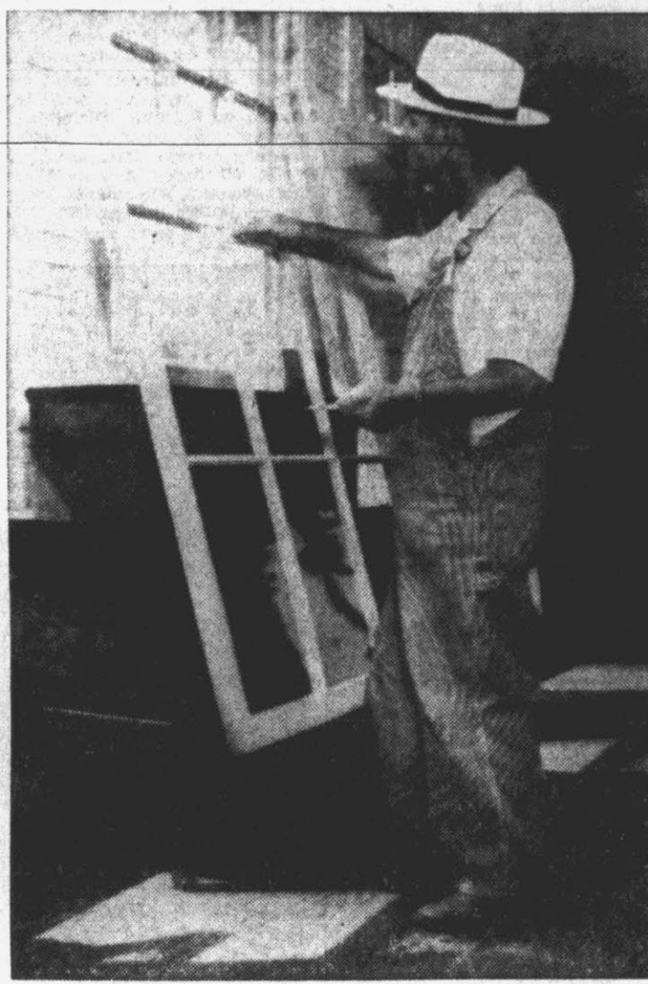
WINDOW DEPARTMENT —Arthur Robinson has made about 60 window sashes this summer for installation in schools throughout the county. Most of the sashes in Pitt's rural schools are odd-sized and maintenance men have it to be quicker and cheaper to make them than to place special orders for them.
