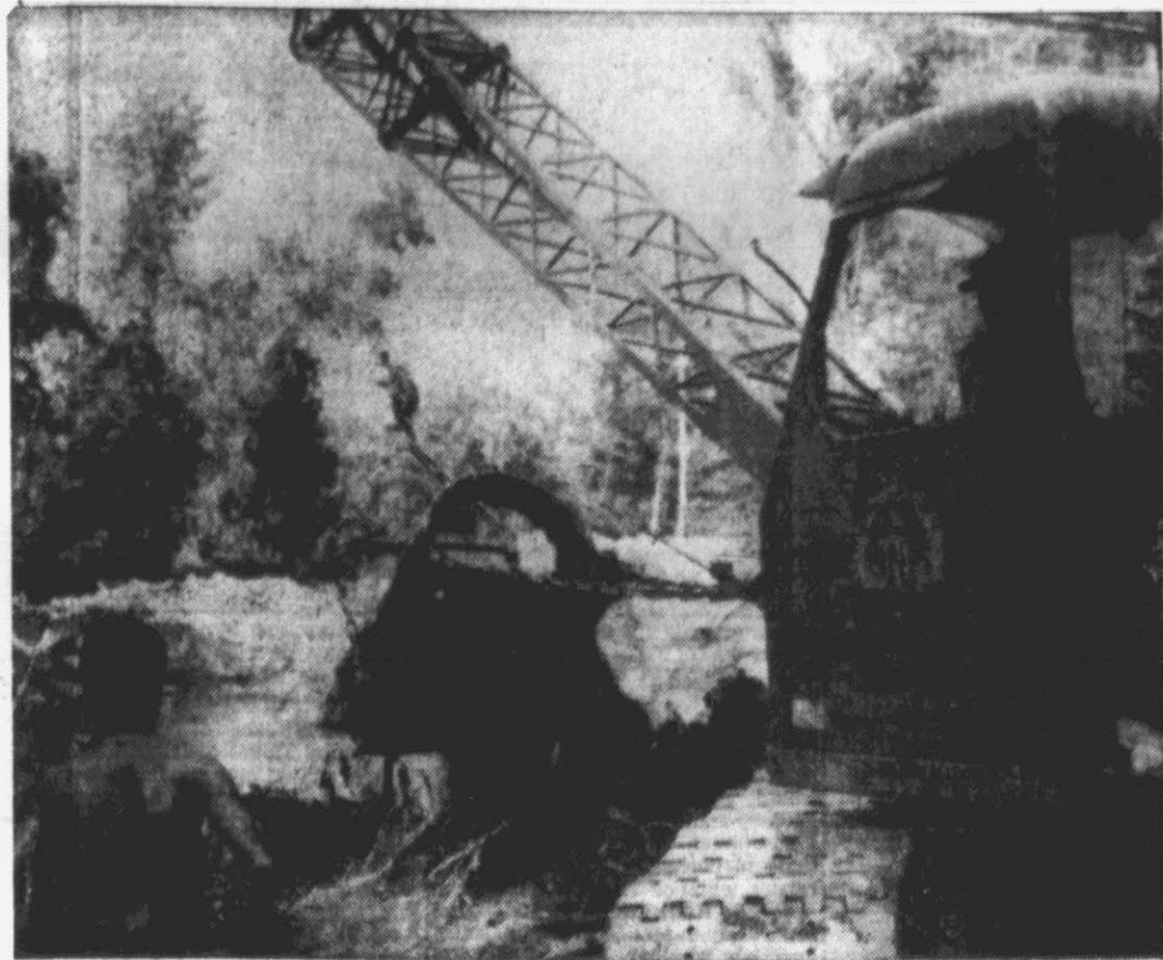
DRAGLINE AT WORK
