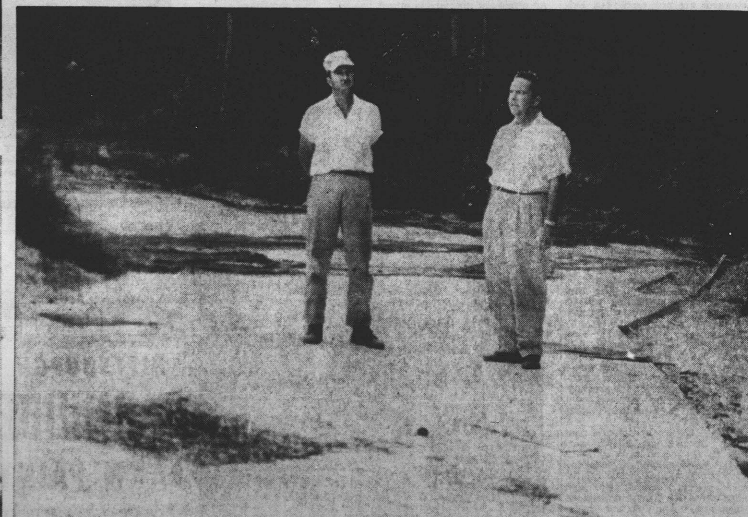
McLAWHORN, WINCHESTER . . . concrete ramp to silos.
