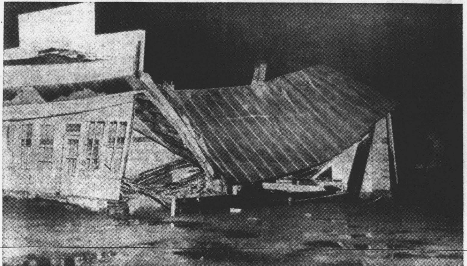
BUILDING TWISTED . . . blown out side narrowly missed dwelling.
