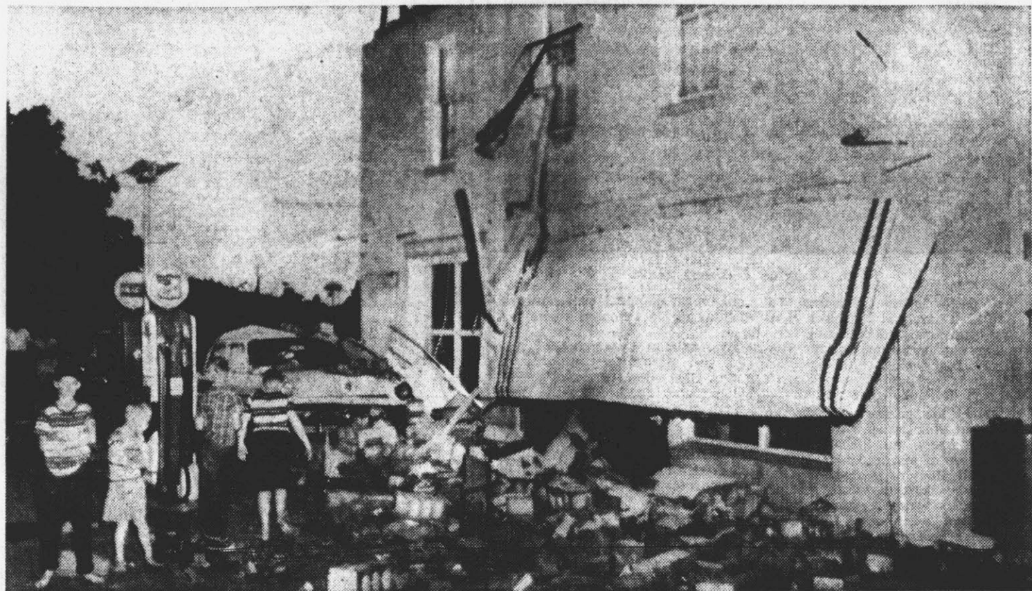
CAR SMASHED . . . winds damaged this building late yesterday.
