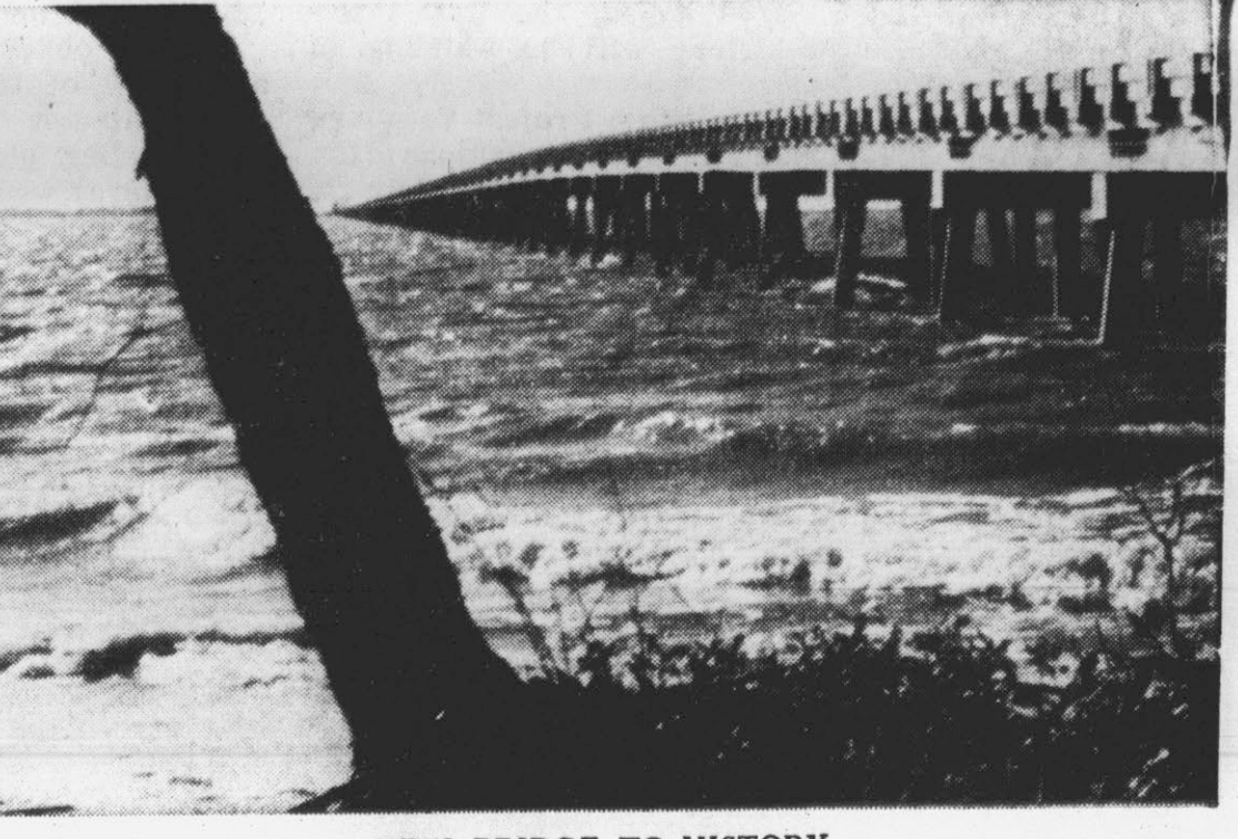
NEW BRIDGE TO HISTORY... Spans Croatan Sound between Manns Harbor and Roanoke Island on U.S 264.
