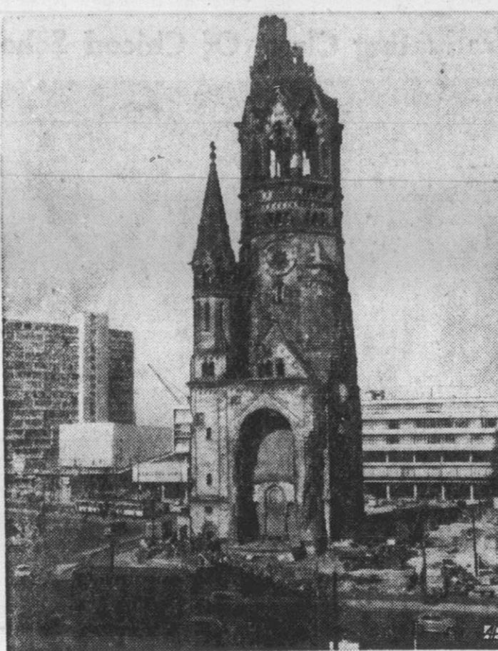
RAZING PROTESTED —Demolition of the war-torn Kaiser Wilhelm memorial church raised protests by West Berliners who want it preserved as "reminder" of World War II.
