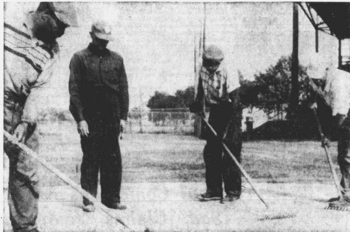
ROUGH SPOTS —These workers are smoothing out the rough spots in the Greenville ballpark's infield. More than 30 loads of dirt has been hauled into the park and leveled off to give the field proper drainage.
