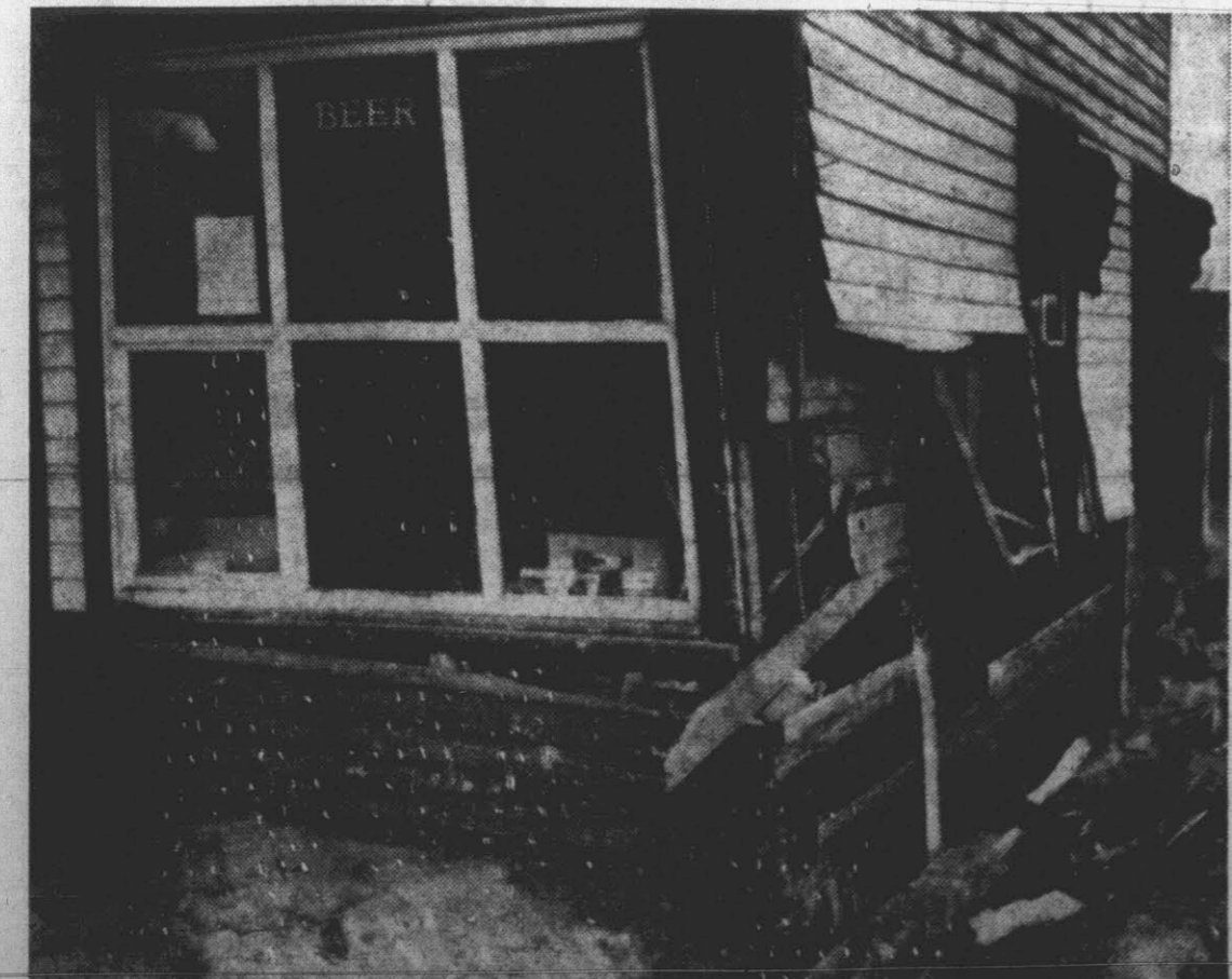
COLLISION—Three men narrowly escaped possible injury yesterday afternoon when a logging truck crashed into the corner of the service station pictured above. The accident took place in Stokes at 2:50 p.m. Patrolman J. B. Surles of the State Highway Patrol estimated the damage to the building at approximately $300. (Reflector Staff Photo).
