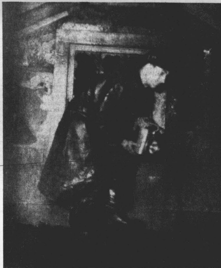
CHECKS BURNED AREA—A fireman above checks a burned area of a dwelling which caught fire around 2:30 last night. Flames burned out the entire second story of the house, located at 613 McKinley Ave. (Reflector Photo by Alvin Taylor).
