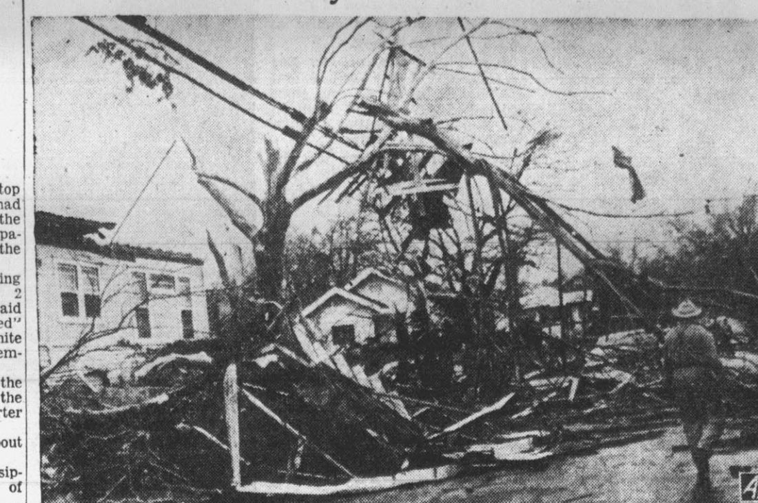
Parts of wrecked buildings, fallen trees and tangled high tension electric wires block a street in Dallas, Tex., after a tornado killed at least nine persons there late Tuesday.
