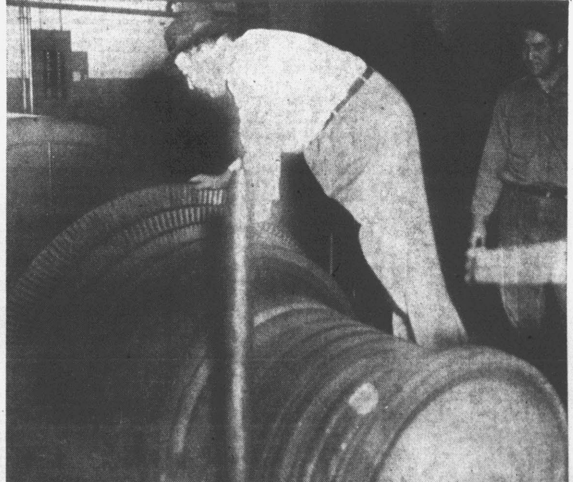
CHECK-UP—Utilities Superintendent Leonard Bloxam takes a look at the blades which, under steam pressure drive the generator. Next week a factory specialist will check the hundreds of blades by tapping each to determine the proper sound. Placing the big cover back in place will be an even harder job since each of the blades wheels fits into its own tight chamber within the top section.
