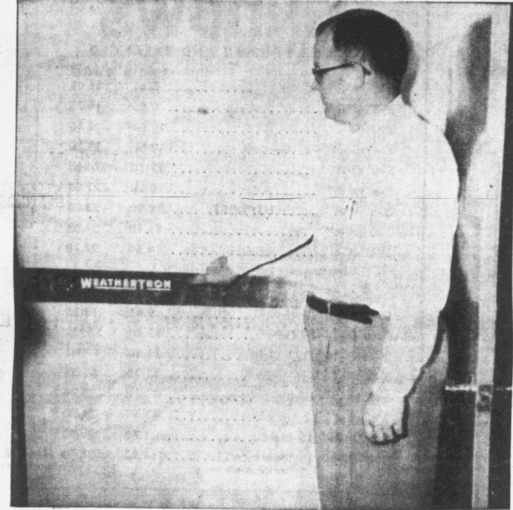
HEAT PUMP—A. B. Goodson, electrical engineer with Greenville Utilities points to a heat pump type heating-cooling unit he installed in his new home. The unit heats and cools by use of compressed gas which is placed under pressure by an electric motor driven compressor. Such devices may be common in farm homes of the future. They may also take care of refrigeration and freezing in the farm home of the future. (Reflector Staff Photo).
