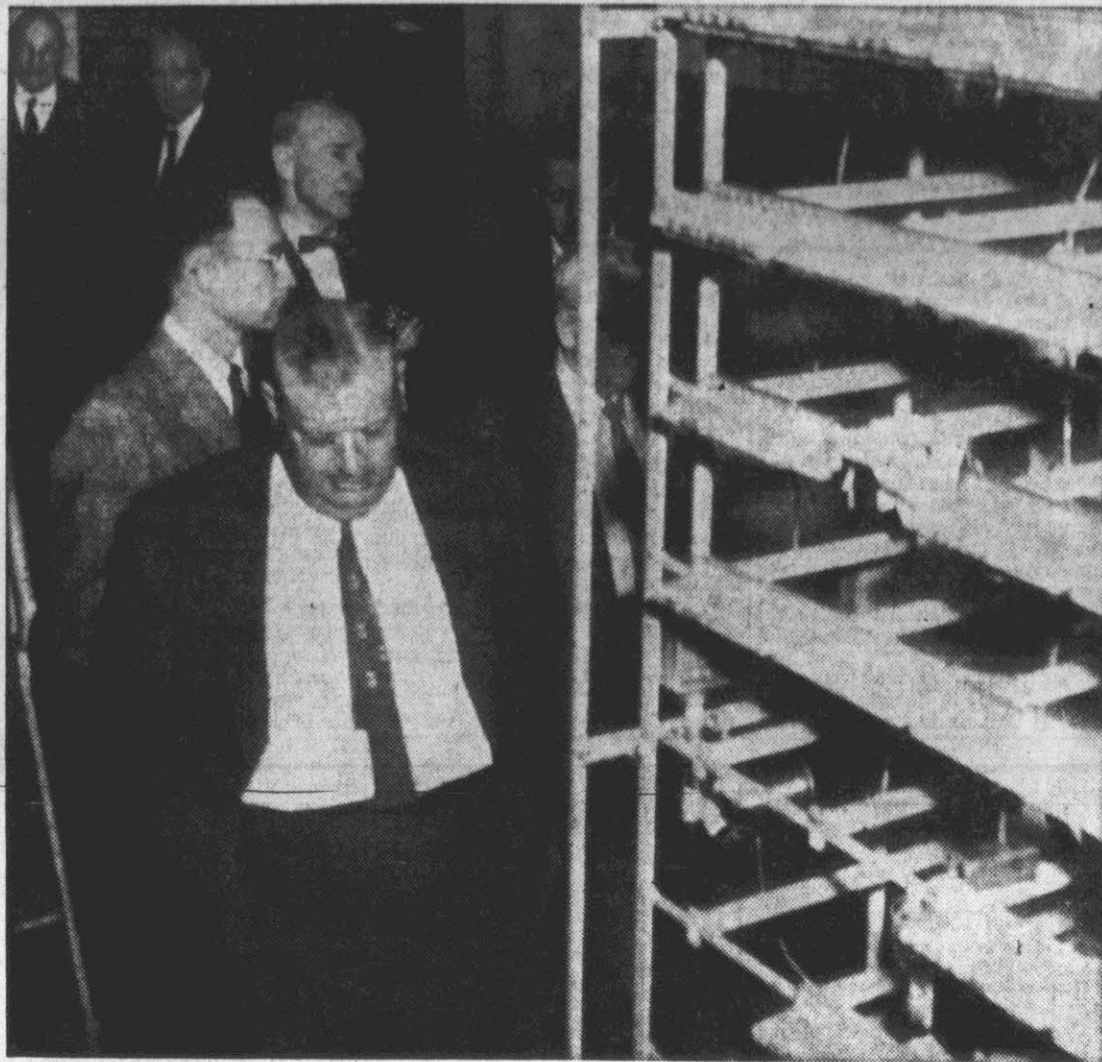
SPECIAL TOUR OF TELEPHONE BUILDING —Looking over equipment in the new Carolina Telephone and Telegraph Company building here are several local business and civic leaders who toured the building Saturday. Guests of the company for Saturday's tour were those who took part in ground-breaking ceremonies for the building 16 months ago. (Reflector Staff Photo).
